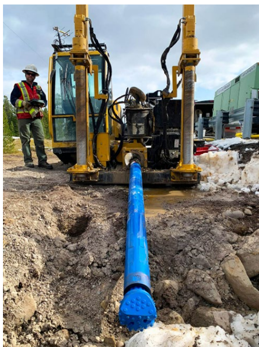
Figure 4.2: Horizontal Directional Drilling Midi Rig
